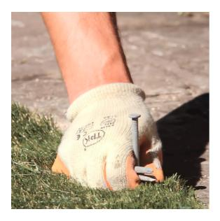
For a clean finish, tuck the artificial grass into the ground to hide the edges. Alternatively, you can spread a layer of concrete around the perimeter (often known as a haunch edge). The concrete should be approximately 50mm deep and 100mm wide with a flat smooth top.
